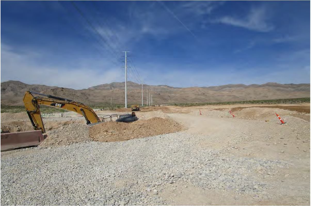
Tropical Parkway view west, western portion of subject SID on right
