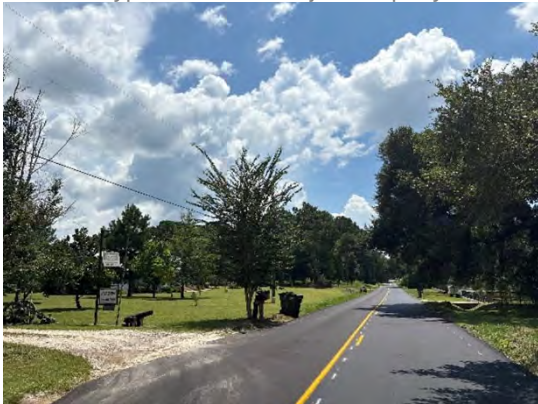
CR 3 Facing South
