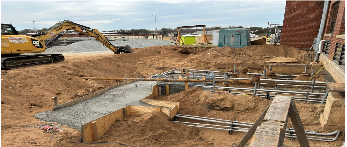
Lower Poplar Influent Pump Station rehabilitation
