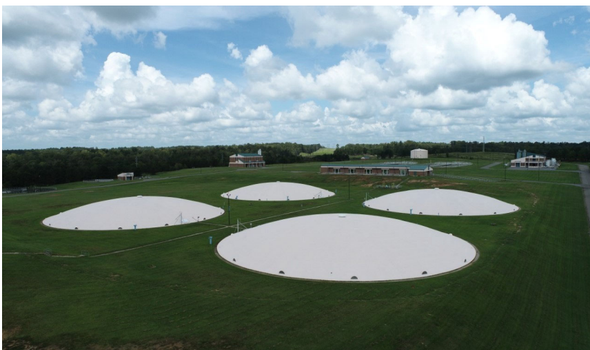
Clear Wells at Frank C. Amerson, Jr., Water Treatment Plant. Each Tank holds 5 million gallons of finished water.
