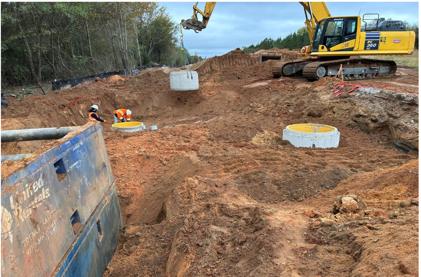
18" Sewer Main rehab
