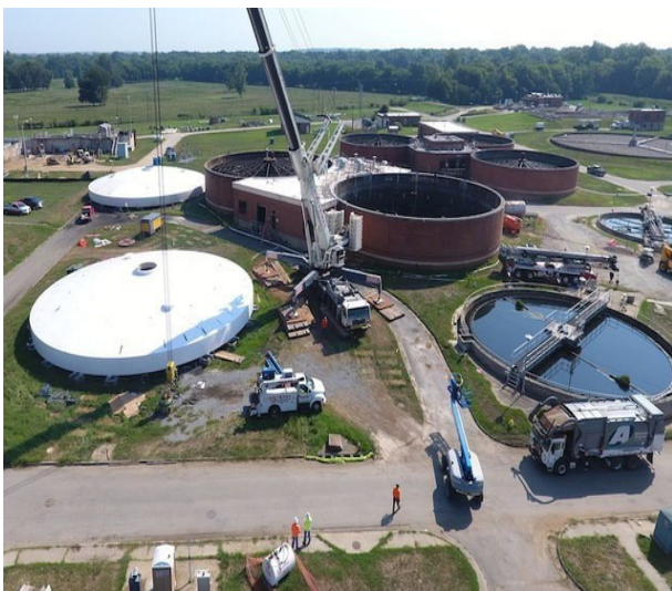
Lower Poplar Digester Lid Replacement
