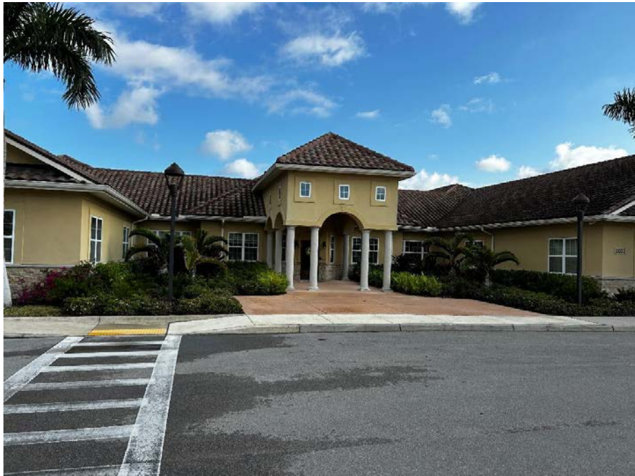
FRONT ELEVATION OF THE SUBJECT IMPROVEMENTS
