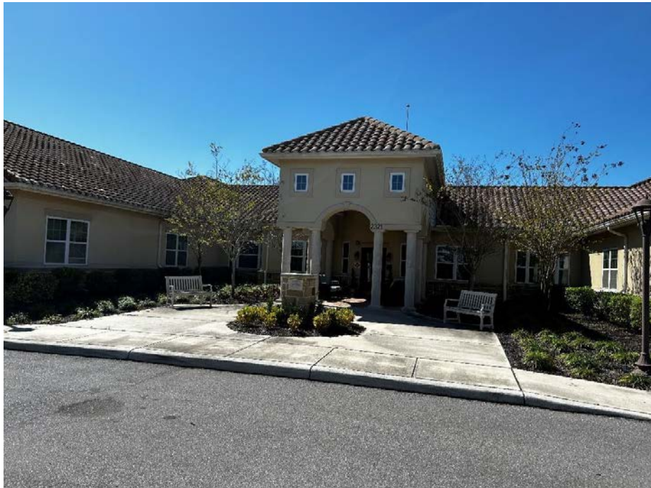
FRONT ELEVATION OF THE SUBJECT IMPROVEMENTS
