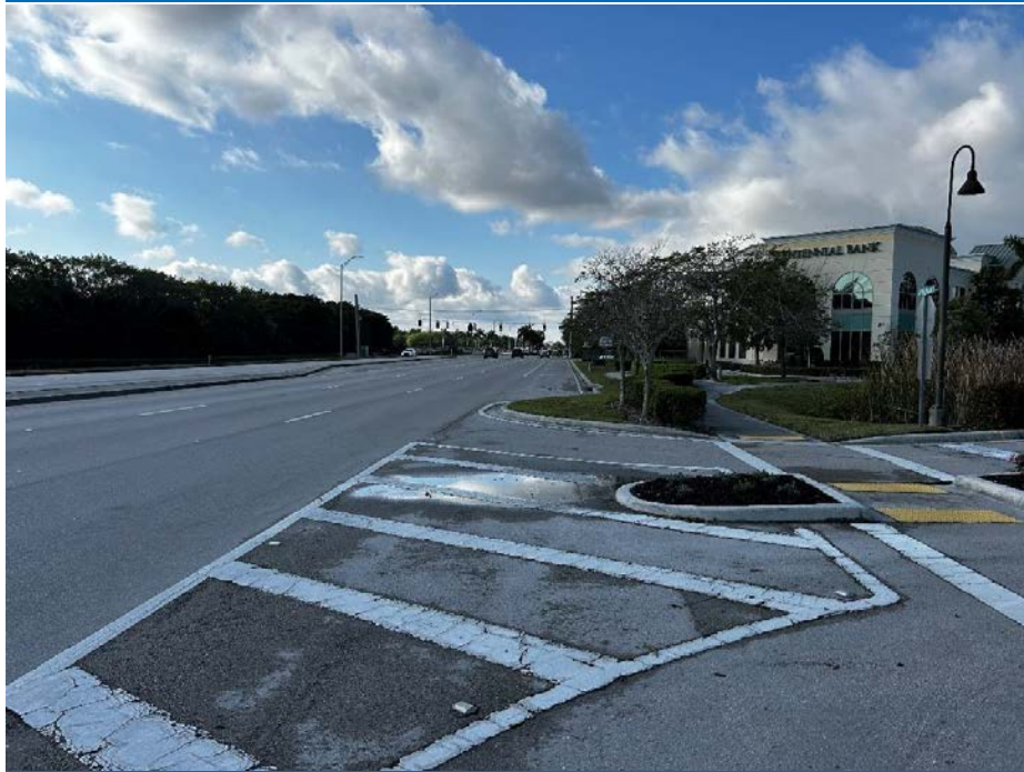
STREETVIEW LOOKING SOUTH ON AIRPORT-PULLING ROAD
