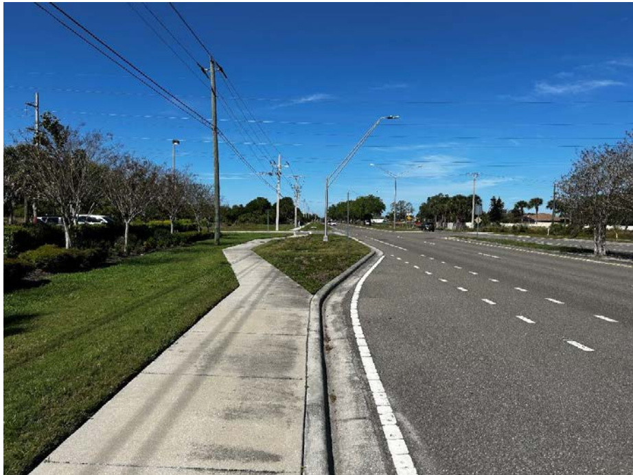
STREETVIEW LOOKING WEST ON EAST VENICE AVENUE
