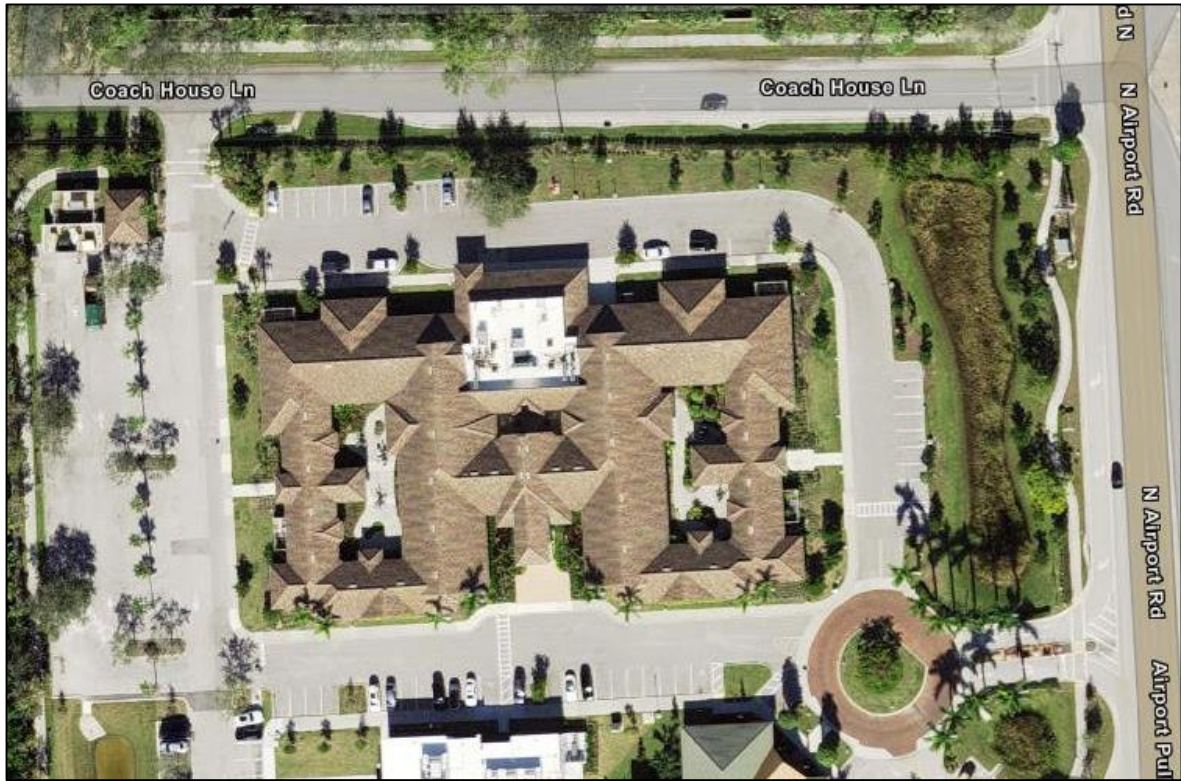
AERIAL PHOTOGRAPH OF THE SUBJECT
