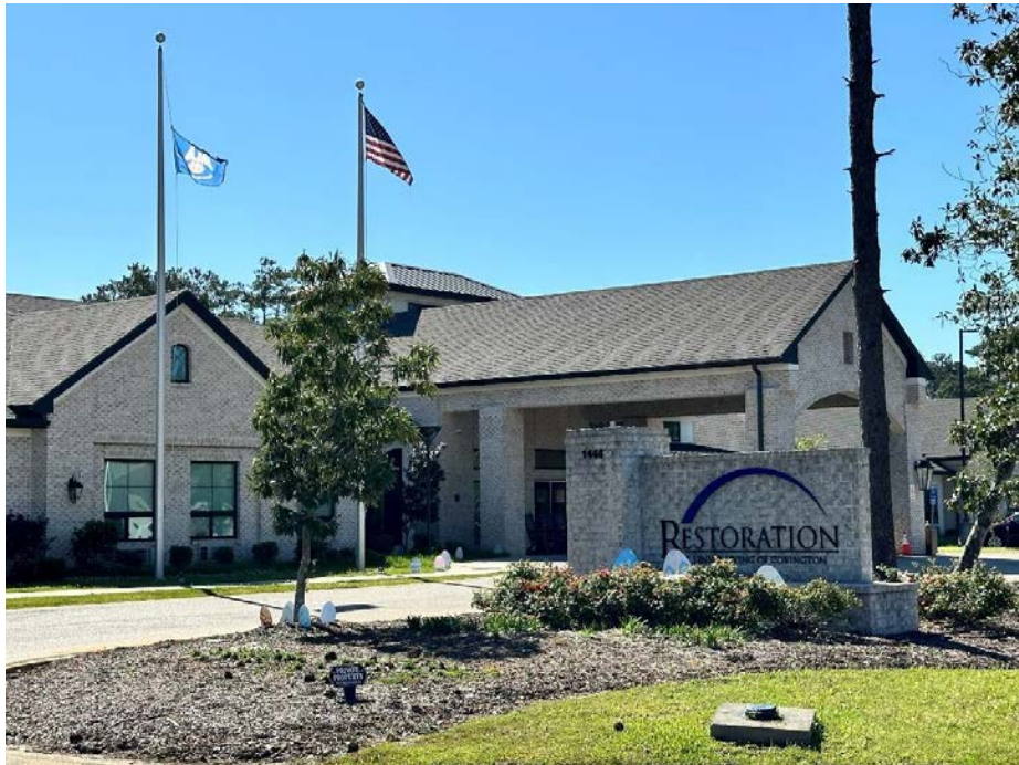
FRONT ELEVATION OF THE SUBJECT IMPROVEMENTS
