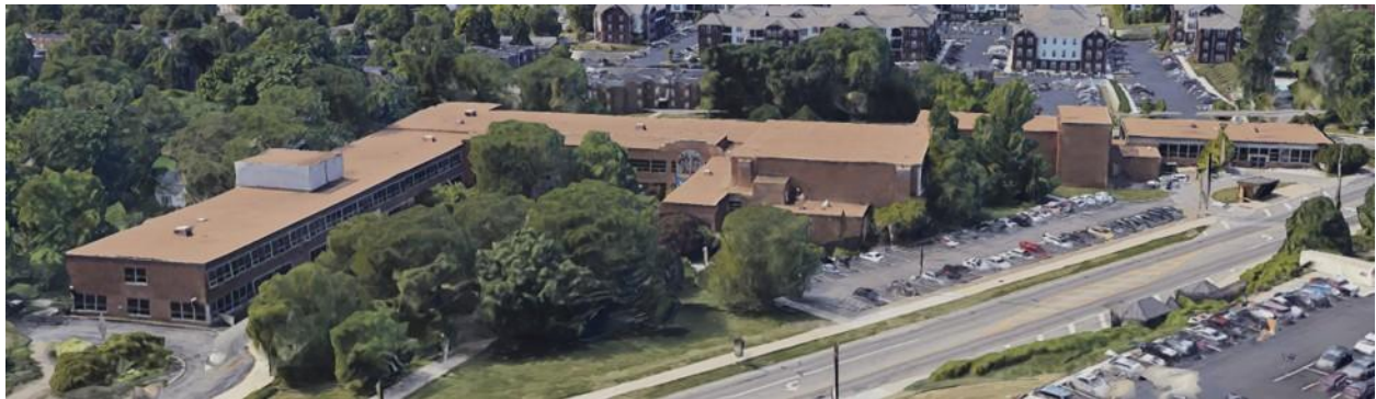
Northern façade of Schwartz Center, with Summit Street in foreground
