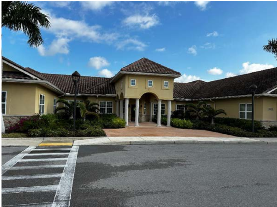
FRONT ELEVATION OF THE SUBJECT IMPROVEMENTS
