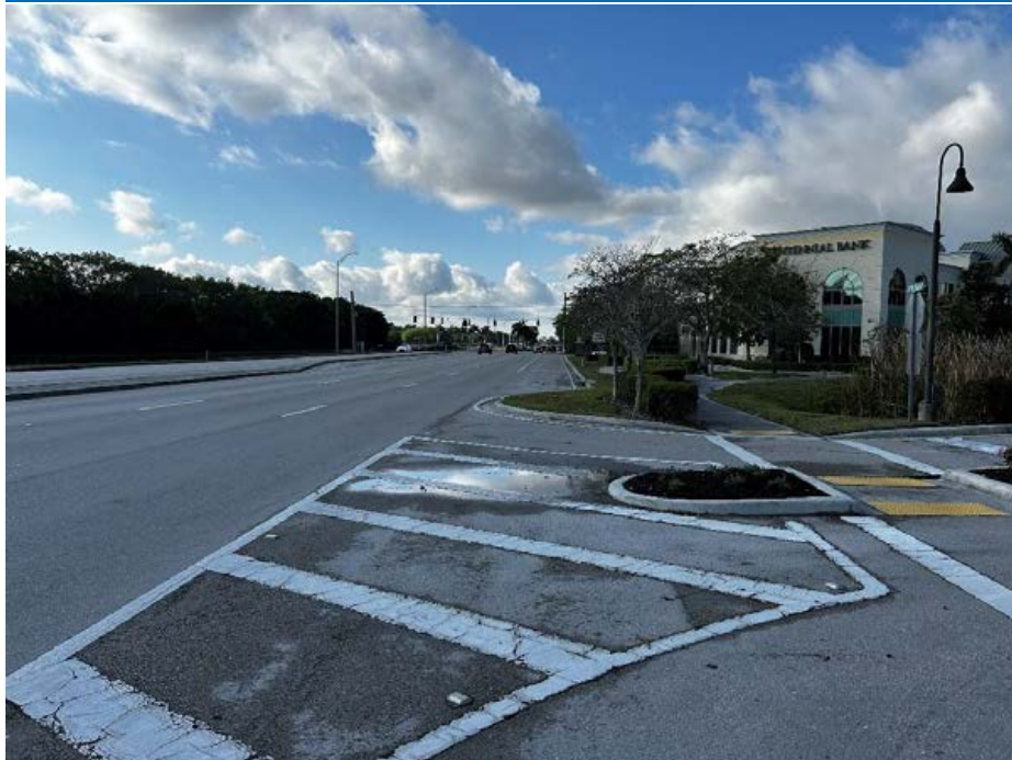
STREETVIEW LOOKING SOUTH ON AIRPORT-PULLING ROAD
