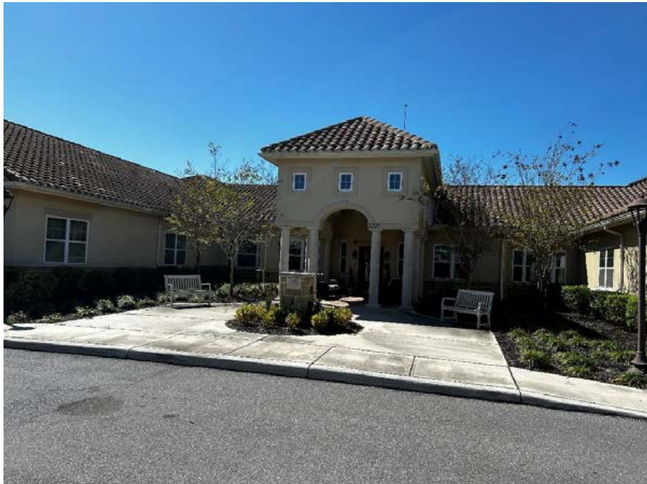
FRONT ELEVATION OF THE SUBJECT IMPROVEMENTS
