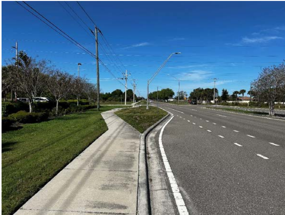
STREETVIEW LOOKING WEST ON EAST VENICE AVENUE
