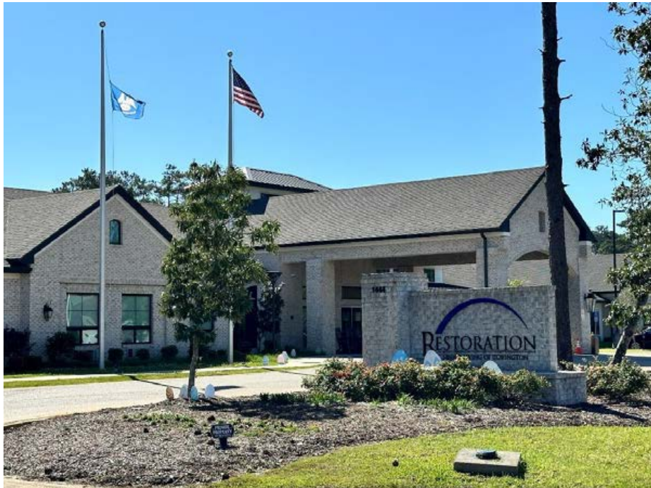
FRONT ELEVATION OF THE SUBJECT IMPROVEMENTS
